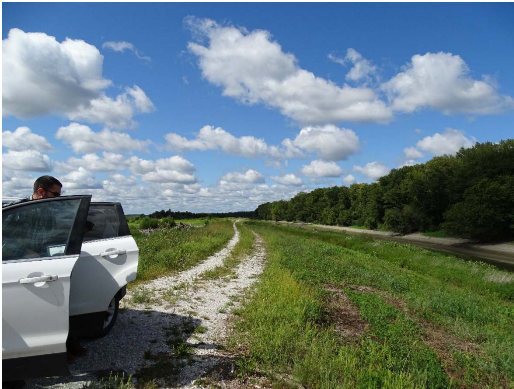
Figure 9: Levee Roadstone (Typical)
