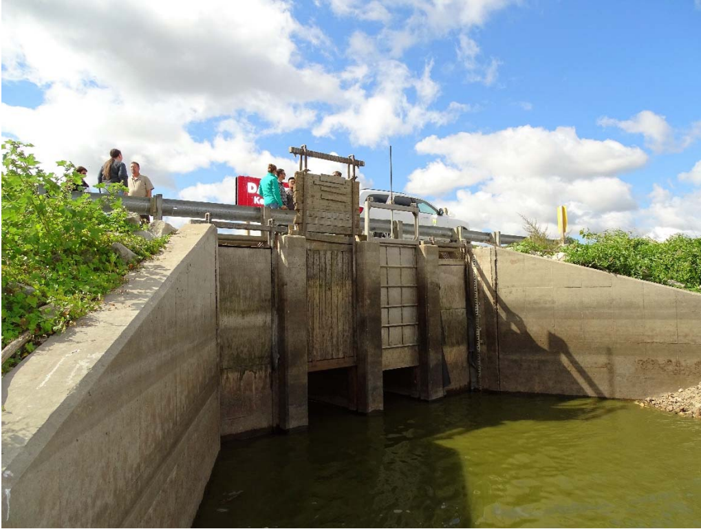
Figure 2: Water Control Structure
