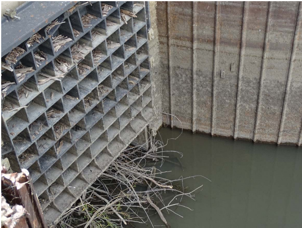
Figure 13: Beaver Intrusion on Cellular Structure
